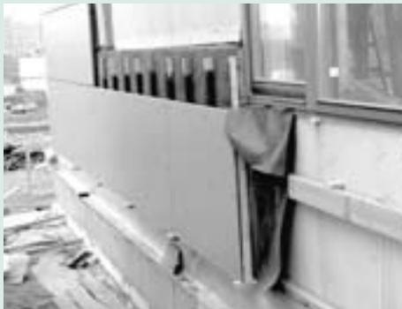
**B<sub>2</sub>) bearing grid from system profiles from aluminum, zinc coated sheets (the systems EuroFox, SPEEDY, SPIDY, etc.)**
