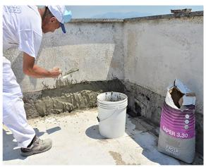
The AQUAZIP ELASTOBAND will be positioned along the connections between the horizontal plane and the vertical overlaps. The strip must be laid continuously on the application surfaces, first applying an at least 2 mm thick layer of AQUAZIP FAST waterproofing membrane, to a width exceeding the strip and making sure to leave the centre part free. For perfect sealing of the corners, use the appropriate preformed elements.
