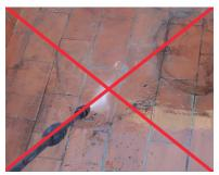
After cleaning, the slope lines must be checked and verified. In fact, any imperfections and/or irregularities present on the substrate, such as dips or depressions, may lead to areas where rainwater stagnates. To repair these areas, treat the surfaces with FASSA EPOXY 400 and then apply GAPER 3.30 before this dries.
