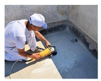
It is recommended not to use a high-pressure washer to clean the old flooring, as this will lead to more water in the underlying substrate.
