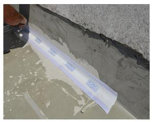
The AQUAZIP fast waterproofing system will also be applied on the vertical overlaps, and after suitable curing will be covered with a coat of KI7 or KZ 35, lime and cement base coat plasters/renders for exteriors and interiors, mixed with a solution of water and AG 15 (1 part AG 15 to 3 parts water), dispersion of synthetic resins for cement-based products. The base coat plaster must be fine-float finished, embedding wide-weave synthetic plaster reinforcing mesh during application.
