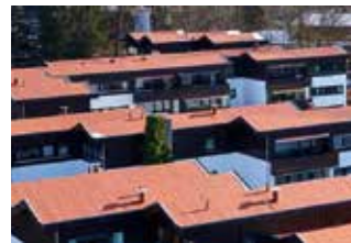
Condominium Oberland, Rhepanol hfk, roof area: 3,300 m 2
