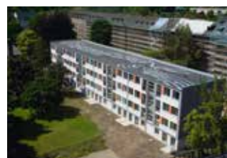
Vivaldi roof painting, Dresden/ Germany, roof area: 870 m 2
