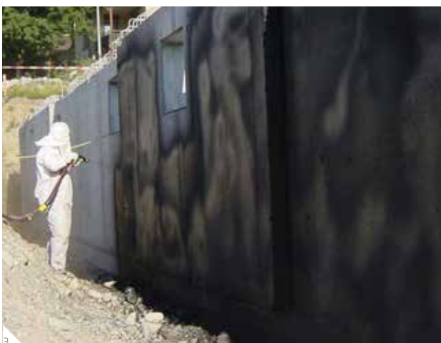
3 Bitumenski premazi in membrane
